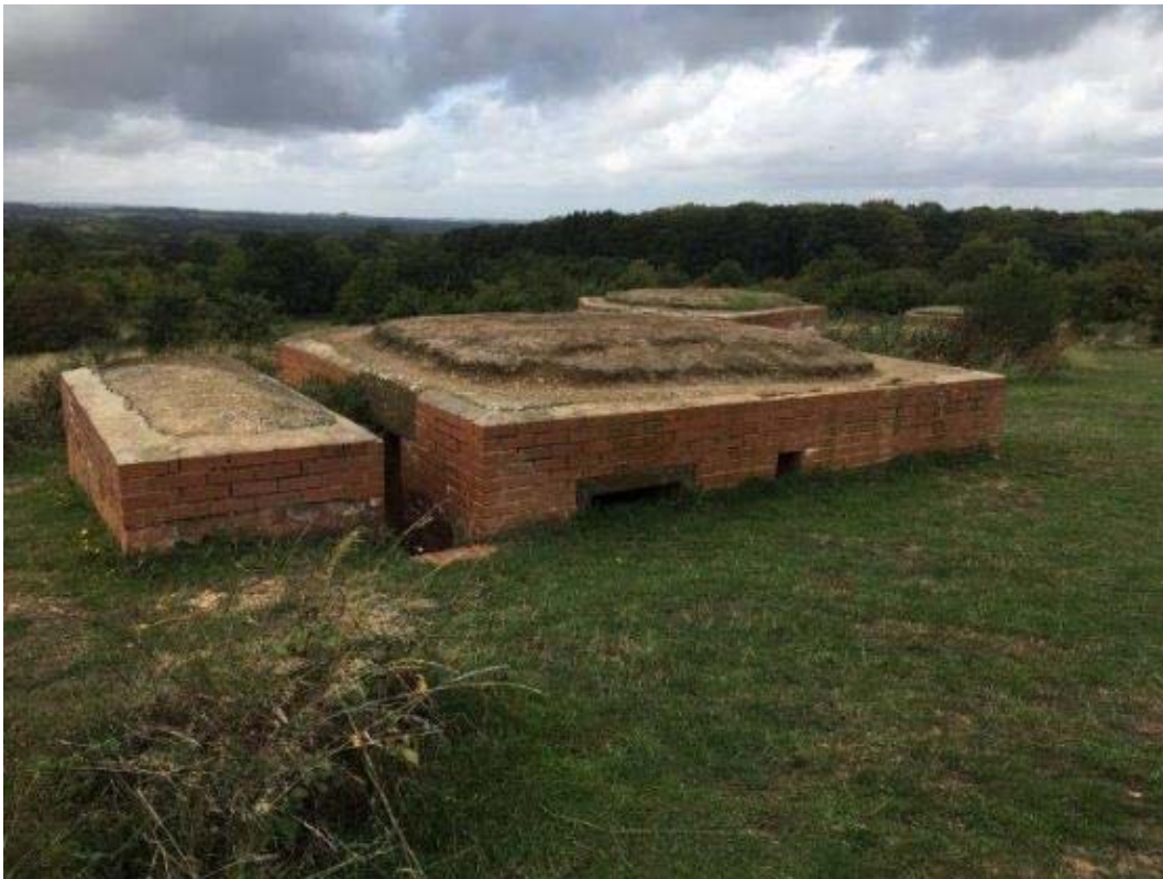
Photograph 9.1.9: WWII Machine Gun Emplacement North West of Ewshot (Asset 631). Taken facing west from NGR SU 81411 50362, 19/09/2018, standard lens.
