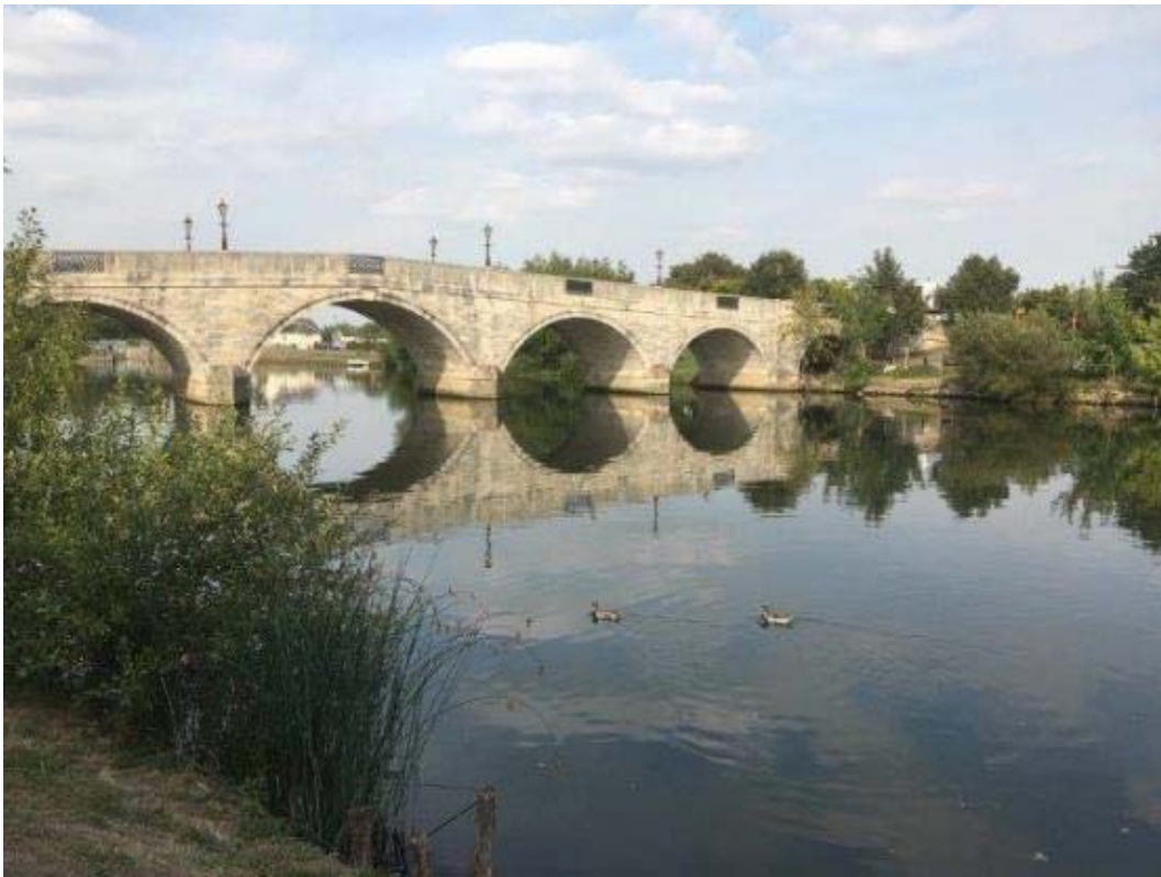
Photograph 9.1.11: Chertsey Bridge (Asset 1035, Asset 1036, Asset 1039). Taken facing north from NGR TQ 05385 66576, 03/09/2018, standard lens.
